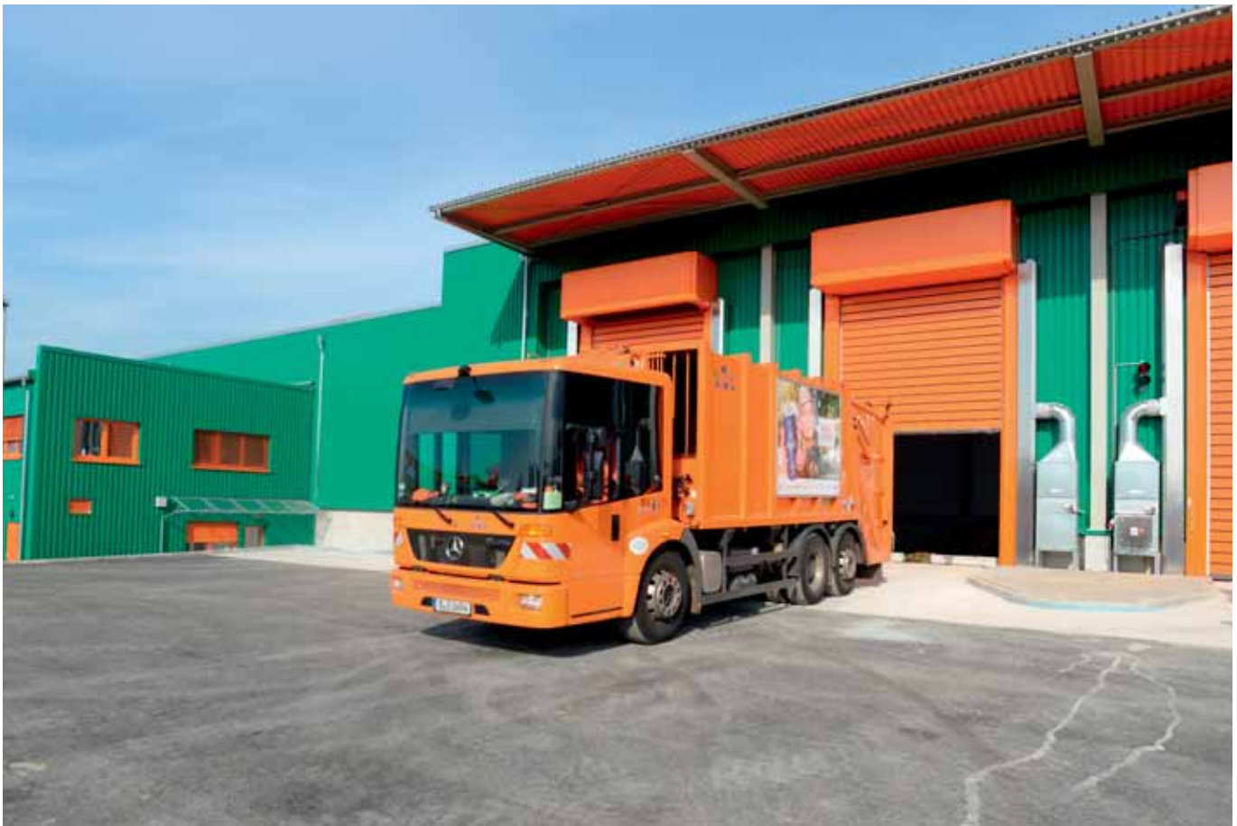
Tipping area of the Ruhleben biogas plant
