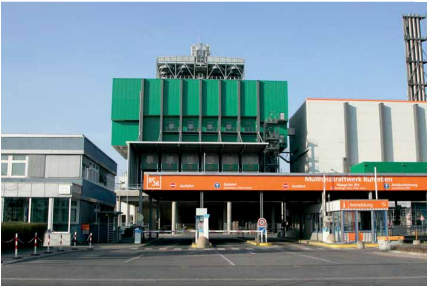
Entrance area of the Ruhleben waste-to-energy power station
