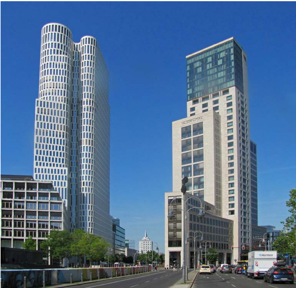
Fig. 8: "Upper West" and "Zoofenster" high-rise buildings on Breitscheidplatz, 2022 (Photo: Kathrin Schellhardt)
