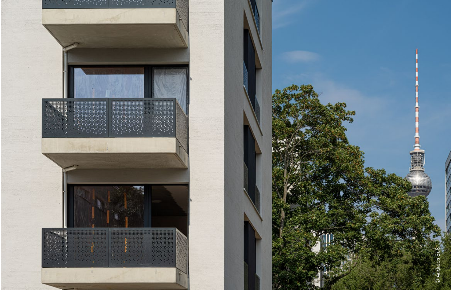
Ifflandstrasse project near Alexanderplatz
