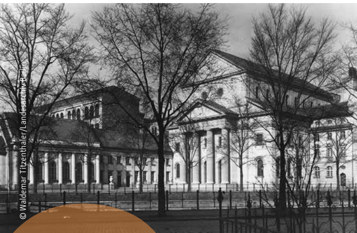
Die Synagoge am damaligen Kottbusser Ufer The synagogue on the former Kottbusser Ufer
