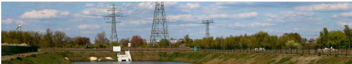
Hochlastsedimentationsbecken (Clean Techn Business Park, Berlin)
