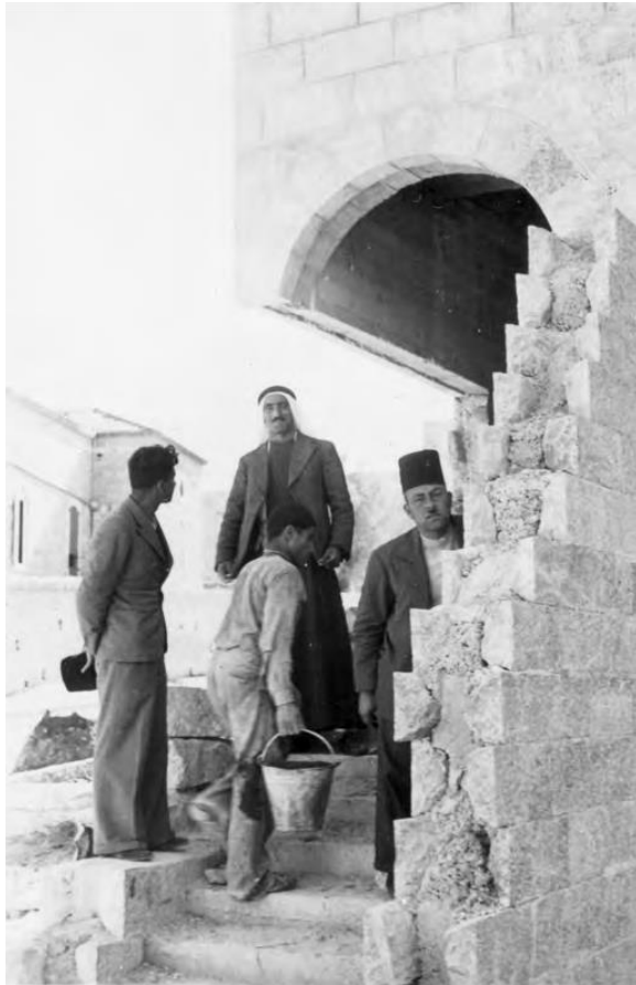
Fig.9. Selmanagić on a construction site in Jerusalem (first on the left). Photo: Selmanagić Archive, Berlin
