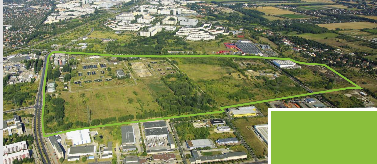
Area plan for the upcoming Clean Tech Business Park Berlin-Marzahn (Photo: Stefan Otto – Aperçu Verlagsgesellschaft)
